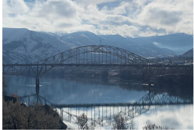
Figure 2-14: George Sellar (SR285) Bridge
